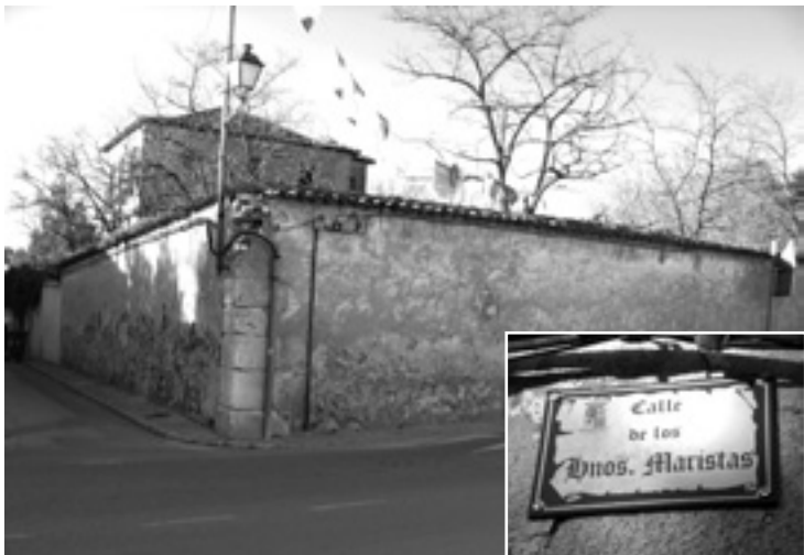
The Brothers' School in Chinchón, not in use anymore but still showing the original structure. The road is now called Marist Brothers Street.
