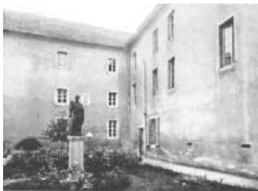
Patio interior de la Capucinière, Belley.
